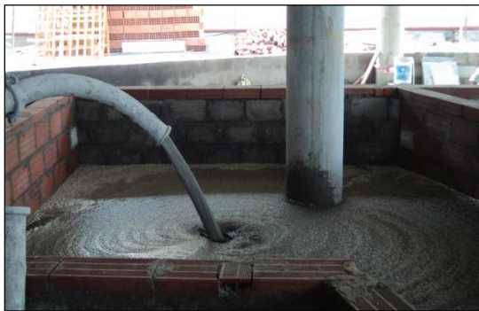
Utility area filling
